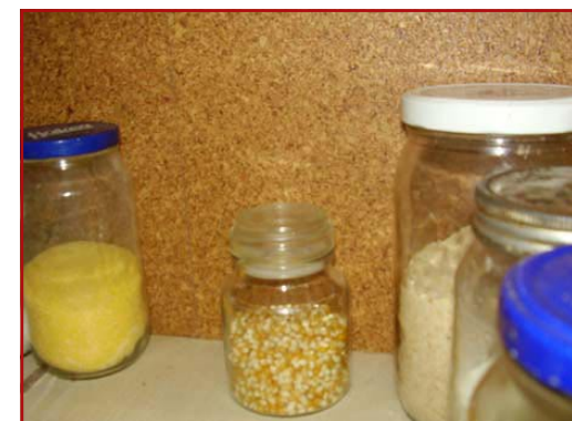
Rear of kitchen cupboard lined with spare cork tiles on exterior wall.
